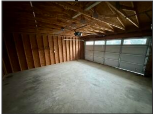
2 Car Attached Garage
